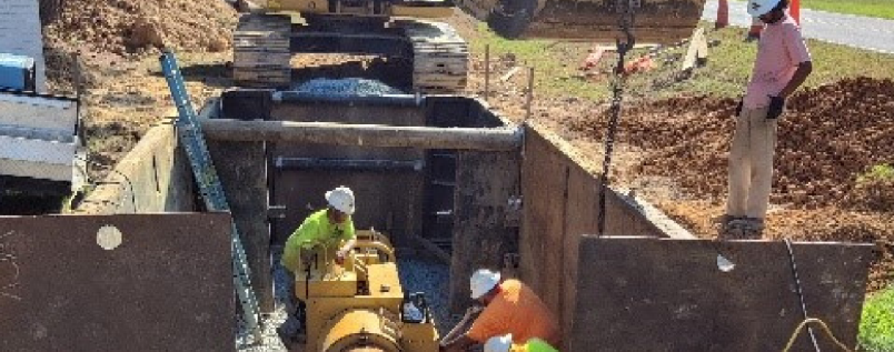
Crews Work Around the Clock on the Waterline Extension
